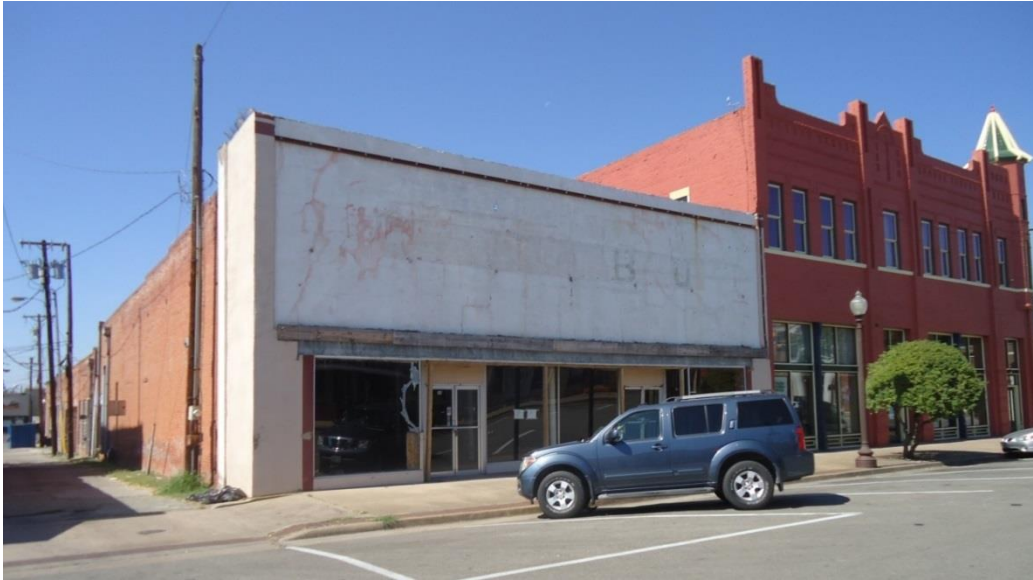
Figure 5: Ben Franklin Store Building, 107 S. Dallas Street, Ennis, Texas, 2015. Building appears to have the same storefront as shown in Figures 2 and 4. The awning was removed a number of years ago after it had deteriorated.
