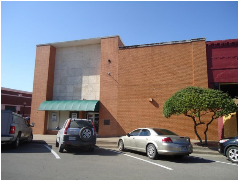
Figure 8: Former Ennis State Bank Building, 113-15 N. Dallas Avenue, 2015. The storefront at 115 N. Dallas Avenue received the new façade prior to 1970.
