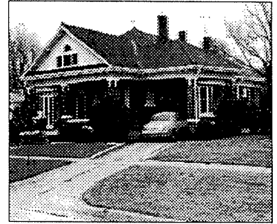
201 N. Gaines (Site No. 761) c. 1915 James S. Sanderson House An intact, well-rendered bungalow form with multiple materials typical of earlier, more elaborate bungalows. With its multiple roof planes, porch proportions and details, this house exemplifies Craftsman bungalow building traditions. Sanderson was listed in the 1925-26 city directory as a farmer. Listed in the NRHP on September 25, 1986.
