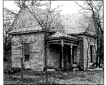
106 E. Denton (Site No. 164) c. 1905 This is a fine example of a modest L-plan dwelling, a house type utilized often in Ennis from the 1880s to the early 1910s. The house retains most of its original fabric and is one of the few to survive with the distinguishing turned posts and porch embellishment intact. Listed in the NRHP on September 25, 1986.
