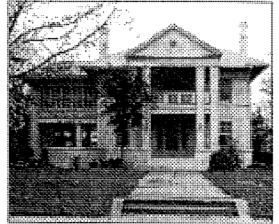
501 N. Preston (Site No. 805) c. 1910 Weatherford House
