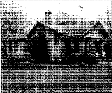
810 N. Preston (Site No. 827) c. 1920 This is one of the most finely crafted and executed local examples of a Craftsman bungalow. The mixture of cladding, triangular braces, multiple-roof planes, cantilevered window bays and porch urns are composed in a prototypical bungalow fashion. Listed in the NRHP on September 25, 1986.
