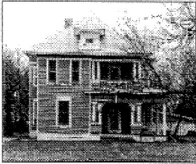
509 W. Brown (Site No. 412) c. 1905 With an asymmetrically-massed composition, more typical of Victorian-era dwellings, this house is adorned with Classical Revival and Craftsman details to create an unusual local variation of early 20th-century eclecticism. Listed in the NRHP on September 25, 1986.
