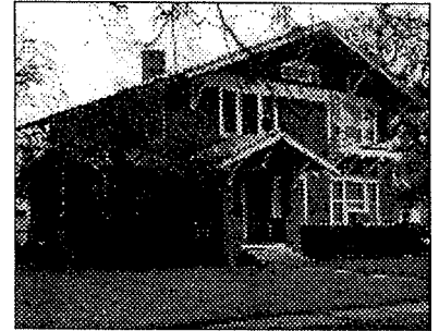
G.G. Dunkerly House (Site No. 258) 1920 607 W. Baylor
