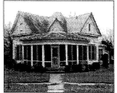
807 N. Preston (Site No. 797) c. 1905 This house illustrates an unusual local variation of a modified L-plan house, the region's most prevalent plan type. Placed on a bias of 45 degree angle to the street, the primary entry at the intersection of two equally massed ells is marked by a decorative gable and five-bay curved porch. This was the home of Dr. W.E. Campbell, a physician and surgeon, who maintained his office at the Moore Building on N. Main Street. Listed in the NRHP on September 25, 1986. .
