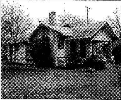
810 N. Preston (Site No. 827) c. 1920 This is one of the most finely crafted and executed local examples of a Craftsman bungalow. The mixture of cladding, triangular braces, multiple-roof planes, cantilevered window bays and porch urns are composed in a prototypical bungalow fashion. Listed in the NRHP on September 25, 1986.
